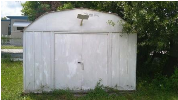
View of old metal shed in the backyard
