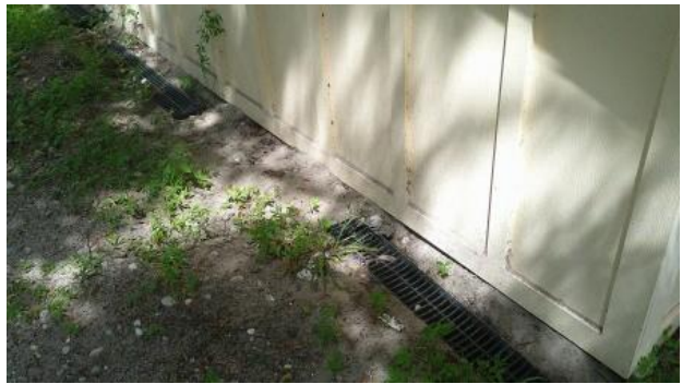
View of French drains installed along part of west elevation of the home
