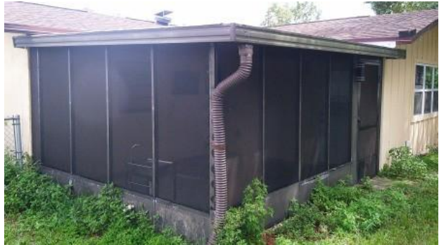
Rear/northwest elevation of subject home
