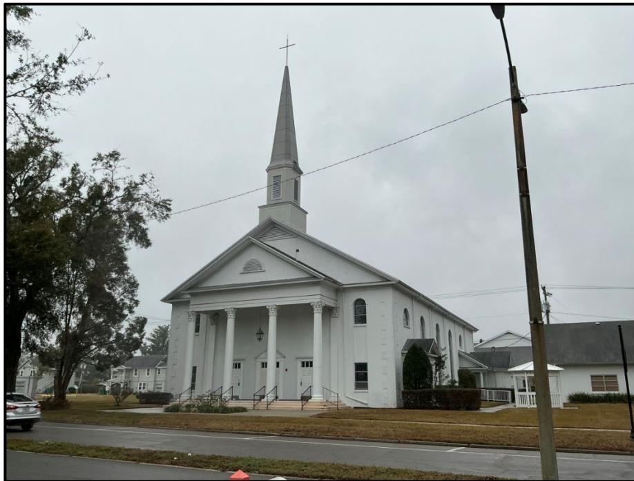
Photograph67. 38635 5th Avenue; recommended contributing (adjacent to Downtown District).
