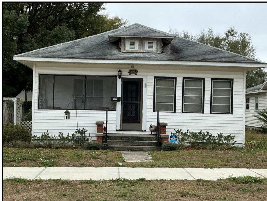
Photograph 20. 5443 9th Street; note vinyl siding, infilled front porch, and replacement windows (recommended noncontributing).
