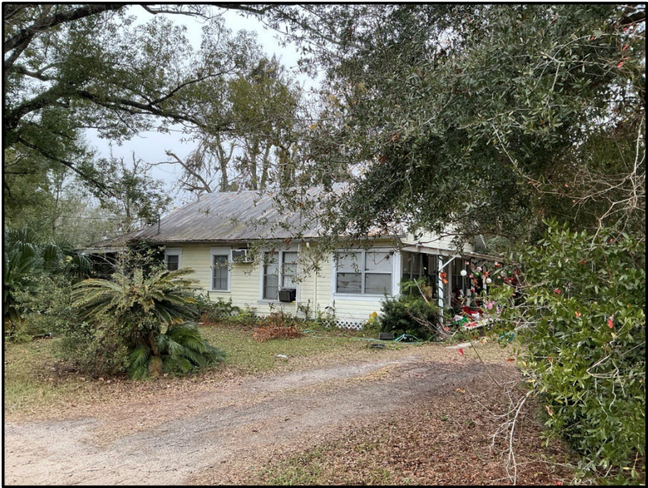
Photograph 22. 5509 9th Street; note front porch enclosed fewer than 50 years ago (new porch added after) and replacement windows not fitting original openings (recommended noncontributing).
