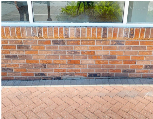
Image 3: Masonry patch material.
