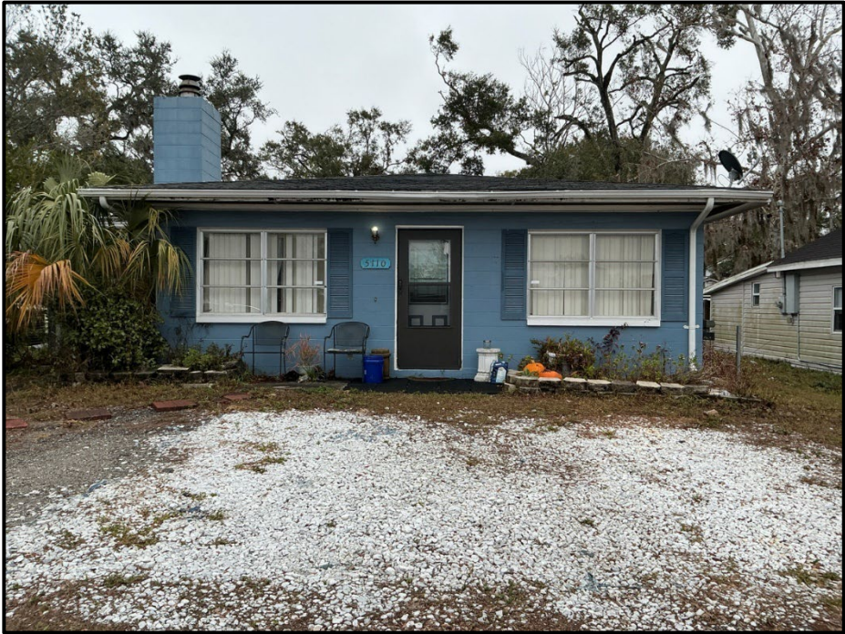
Photograph 9. 5110 7th Street; recommended contributing (adjacent to the Downtown District).
