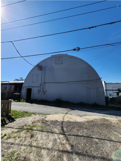
Image 1: North Elevation of Quonset Hut
