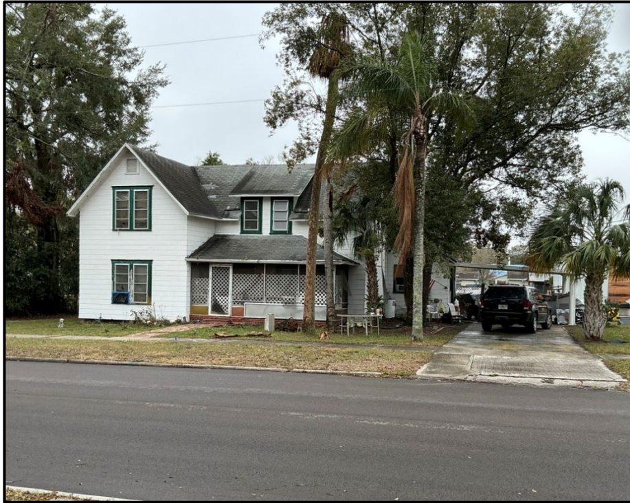
Photograph 11. 5047 8th Street; note incompatible replacement windows and non-historic carport (recommended noncontributing).
