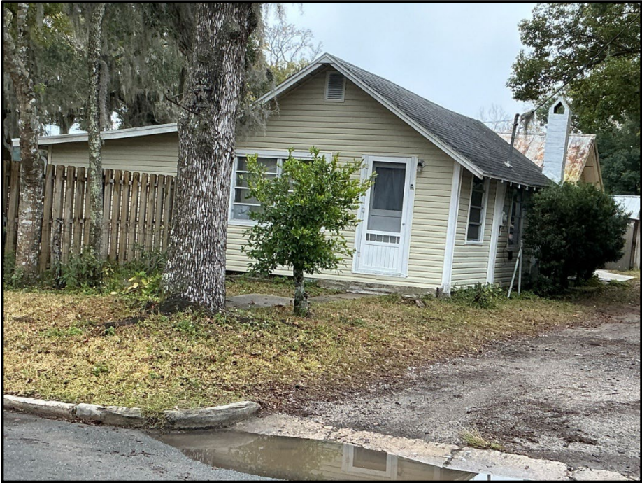
Photograph 1. 38540 4th Avenue; note vinyl siding and large side addition (recommended noncontributing).
