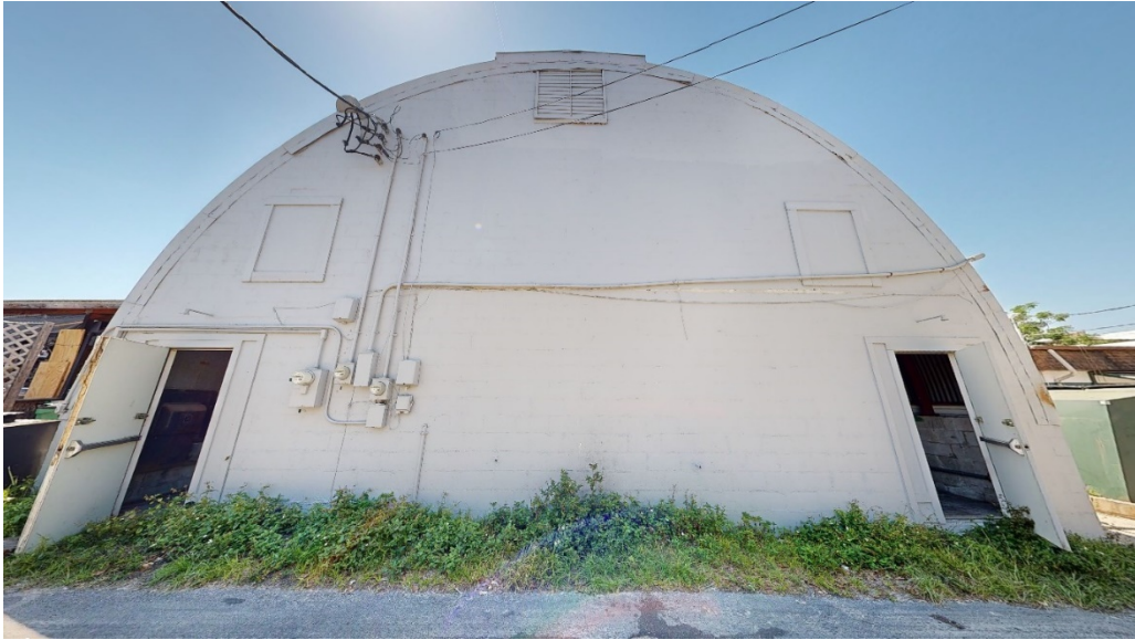
Image 19: Wrapping of corrugated metal material at rear of theater.
