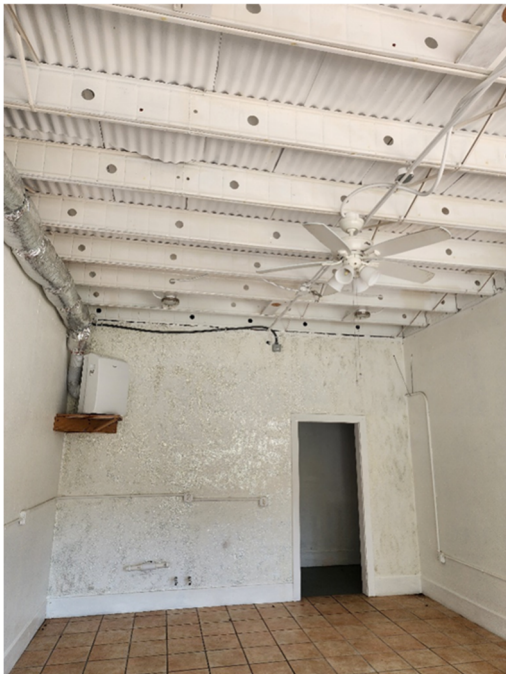
Image 8: Retail 2 Area. Second Floor framing above.
