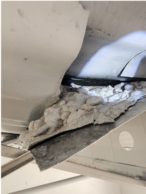
Image 12: Metal/Formwork Decking, slipping from formwork.
