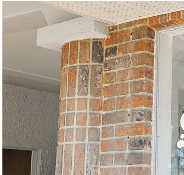
Image 8: Anchor point cavities.
