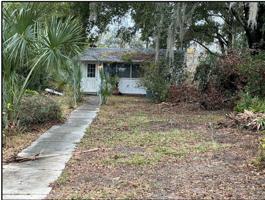
Photograph 12. 5117 8th Street; recommended contributing.
