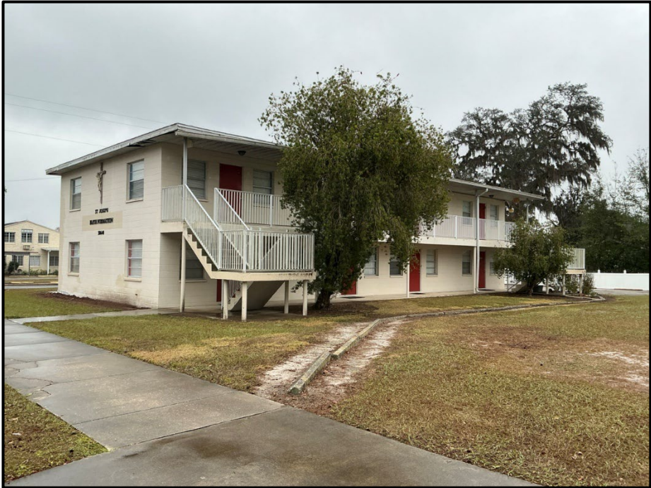
Photograph 7. 38640 5th Avenue; recommended contributing (adjacent to Downtown District).
