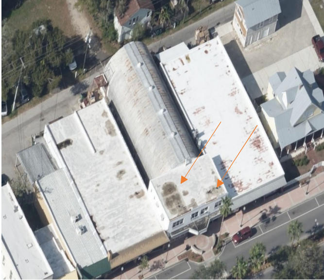
Image 21: Roof stains visible on membrane roof.
