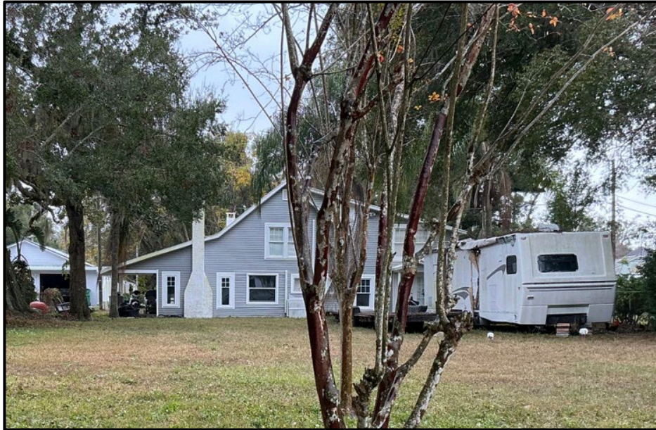
Photograph 35. 5519 11th Street; note vinyl siding and replacement windows (recommended noncontributing).
