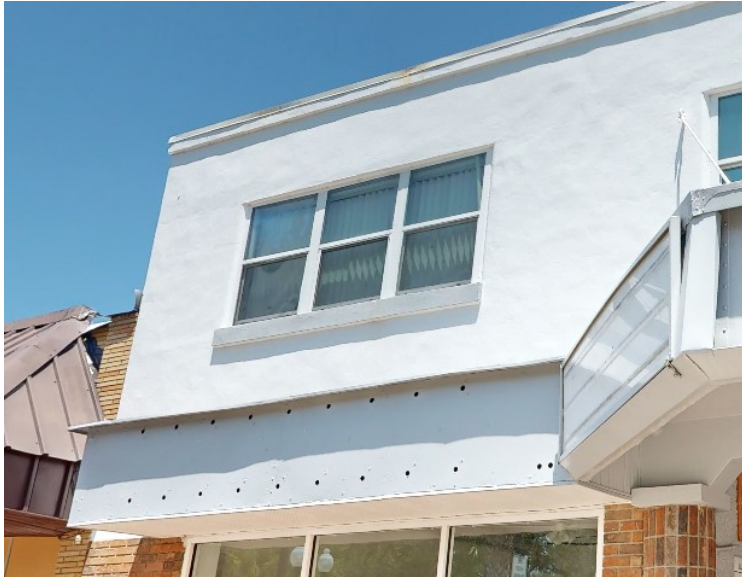
Image 15: Smooth second floor stucco finish.
