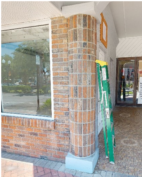
Image 7: Brick coursing at column.
