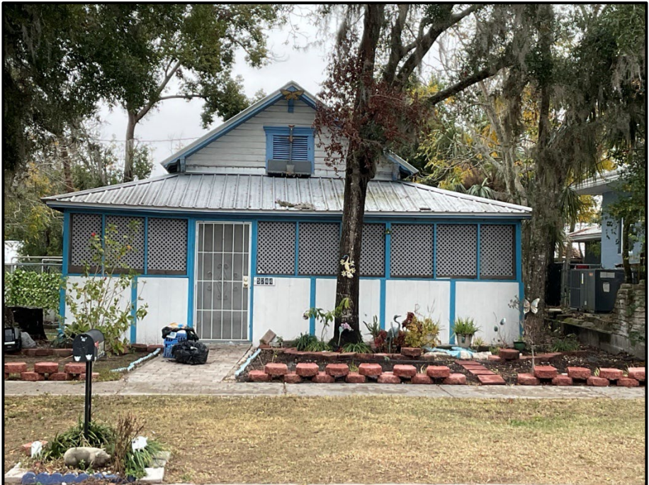
Photograph 18. 5244 9th Street; note enclosed front porch c. 2020 (recommended noncontributing).
