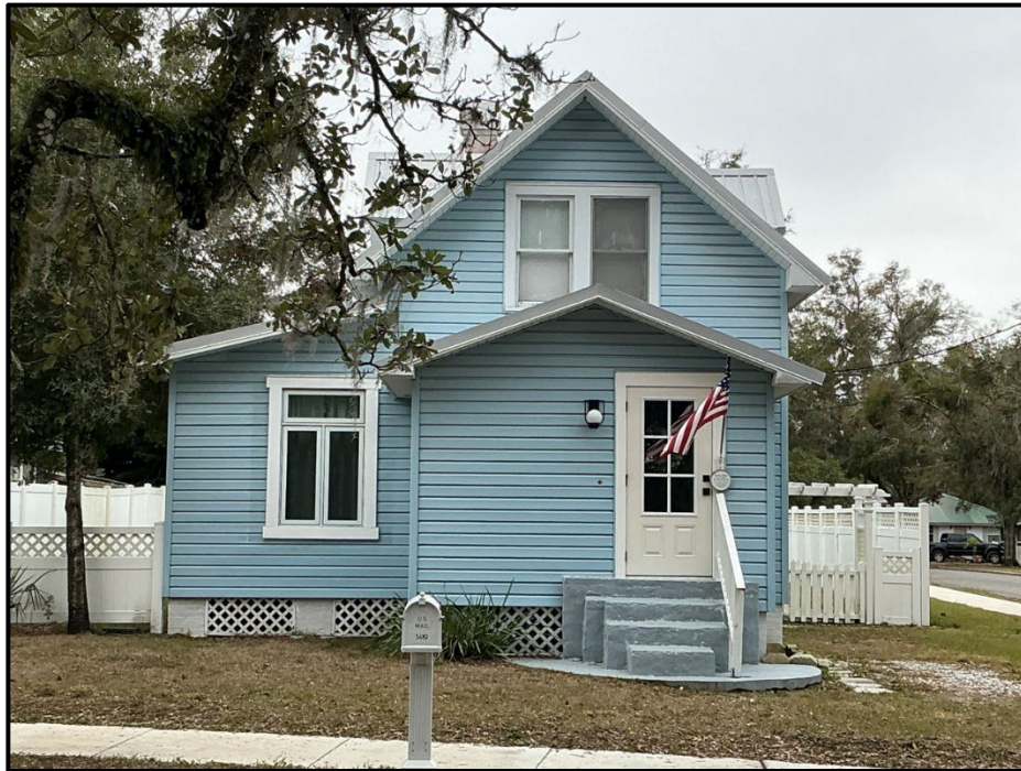
Photograph 19. 5419 9th Street; note vinyl siding, incompatible replacement windows, enclosed front porch, and incompatible front steps (recommended noncontributing).
