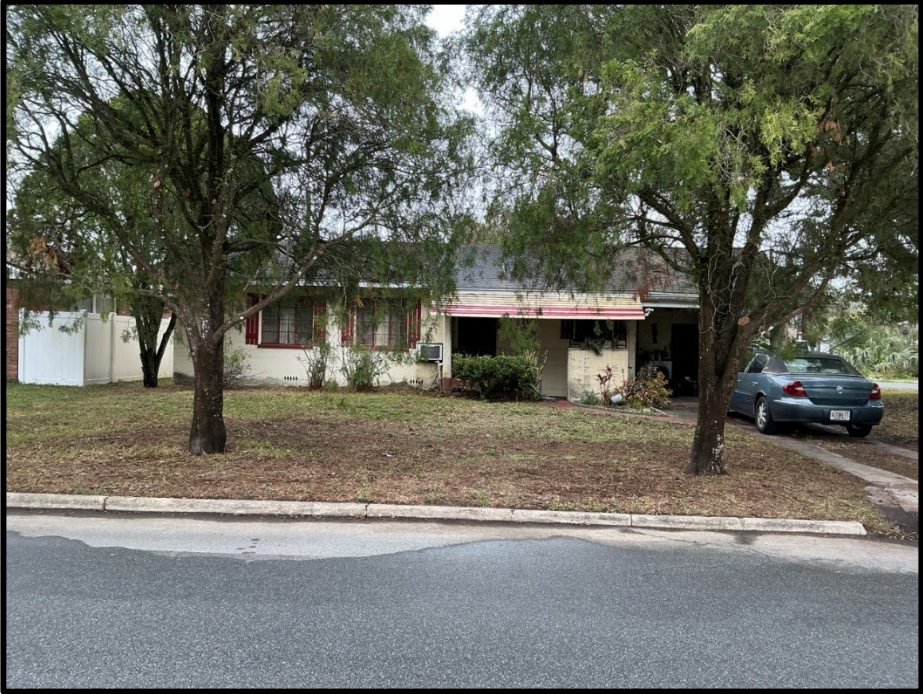
Photograph 29. 5426 11th Street; recommended contributing.
