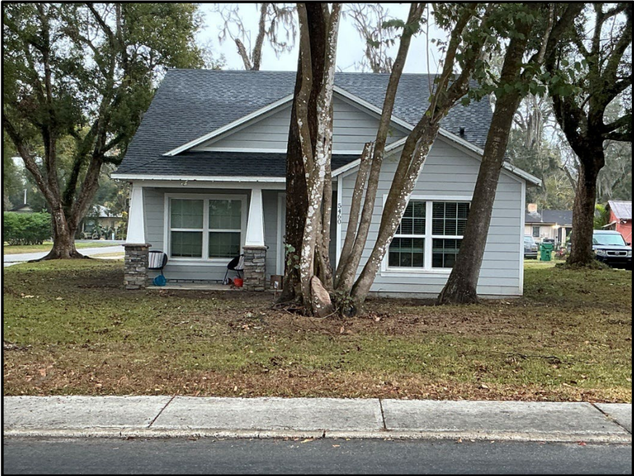
Photograph 31. 5460 11th Street; new construction (recommended noncontributing).
