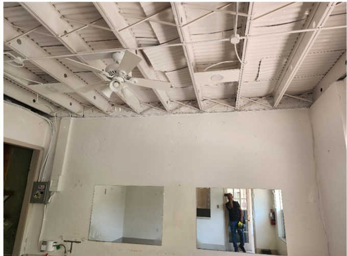
Image 9: Retail 1 Area. Second Floor framing above.
