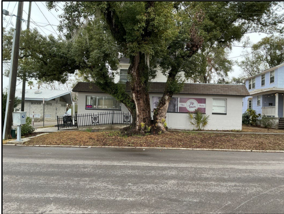
Photograph 13. 5232 8th Street; note obtrusive front additions and replacement windows (recommended noncontributing).
