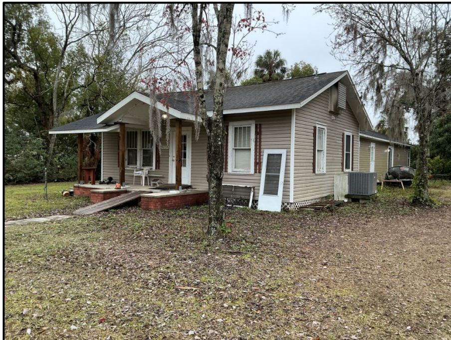
Photograph 14. 5429 8th Street; note vinyl siding, replacement porch posts, and large rear addition (recommended noncontributing).
