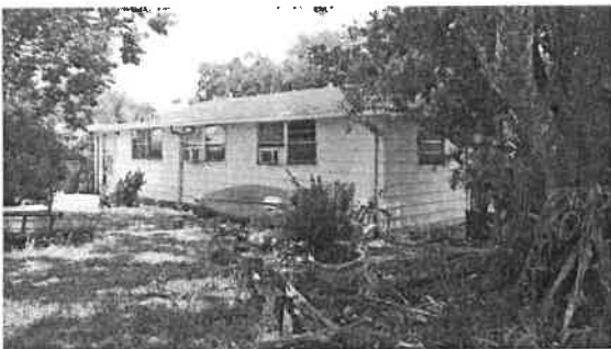
Close-up view of addition in back of the home
