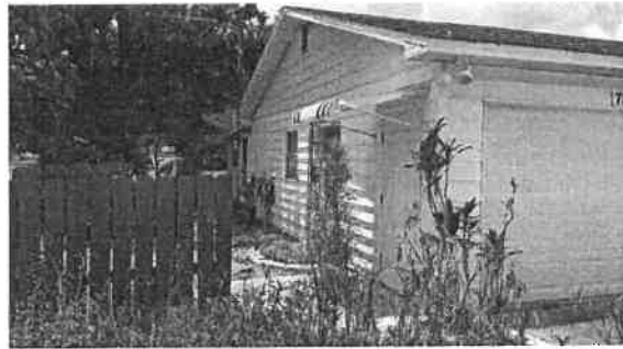
View of west/side elevation of subject home, showing the side garage door
