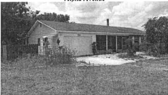
Northwesterly view of front elevation of subject home
