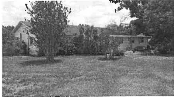
Rear view of subject residence
