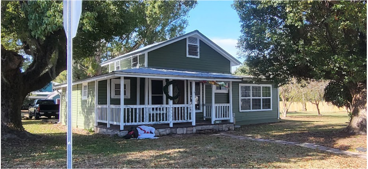
Figure 1 - Current property conditions
