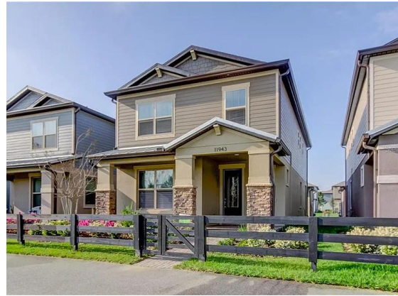
Narrow-lot homes with alley-loaded garages create a compact development pattern that preserves open space in conservation subdivisions.
