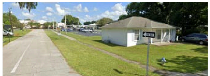
SUB-STANDARD SIDEWALK @ 10TH ST AND SCHOOL
