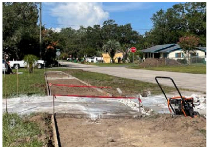
NEW SIDEWALK IMPROVEMENTS
