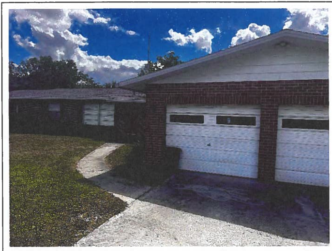
1. View from street facing south.
