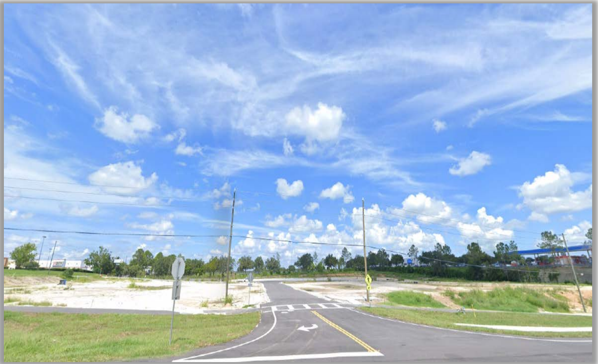
Photo 1 - Project View from Gall Blvd.
