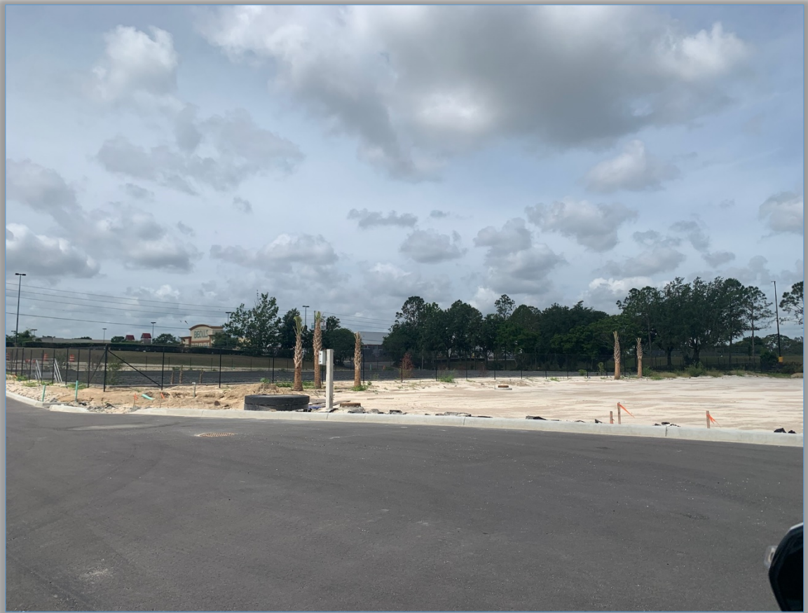
Photo 2- Project Viewed from Interior with Southerly View
