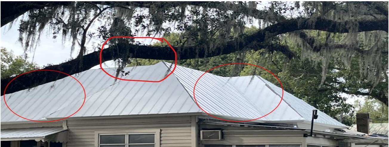
Photo 2 – Alterations (Dormers & Chimney Removed)
