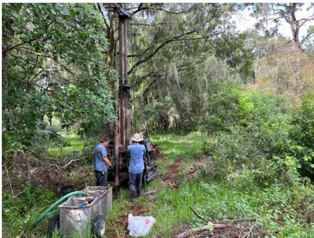
Photograph No. 2: View of soil boring operations at subject property.
