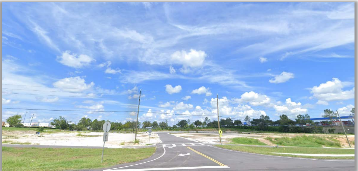
Photo 1 - Project View from Gall Blvd.
