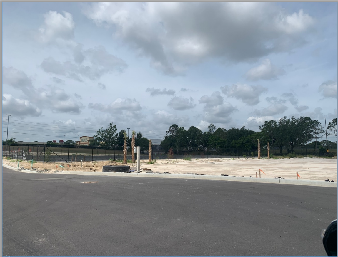
Photo 2- Project Viewed from Interior with Southerly View
