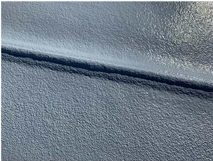
Spray foam and coating over an existing metal roof
