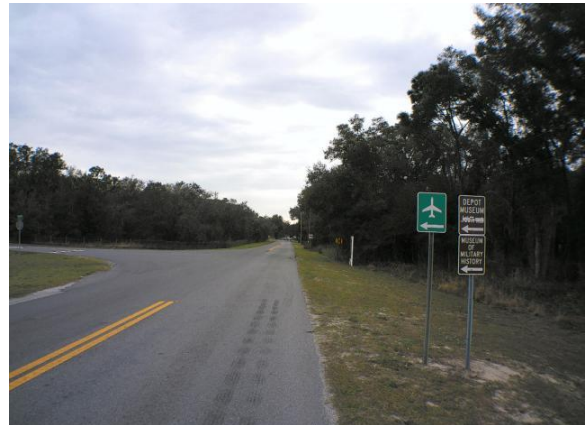
Street Scene: Looking west along 6 th Avenue (Photo Taken on January 26, 2024)
