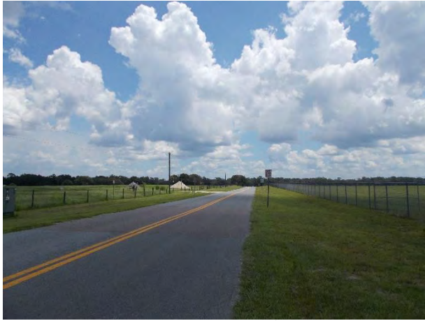
Easterly view along 6 th Avenue
