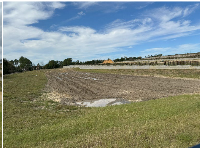
Figure 4b – Retention Pond after de-silting
