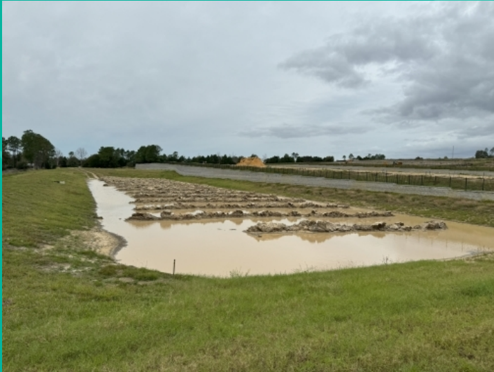
Figure 3a – Pond during de-silting
