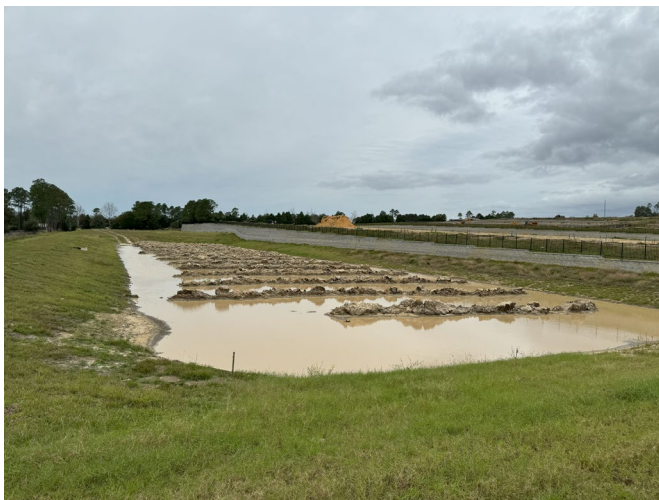
Figure 4a – Retention Pond during de-silting remediation
