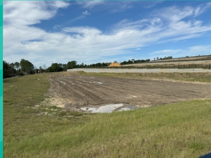
Figure 3b – Pond after de-silting
