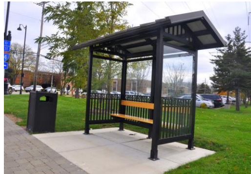
Accessible, sheltered bus stop.
