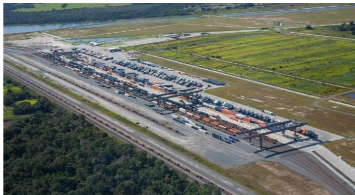
Central Florida Intermodal Logistics Center near Winter Haven.
