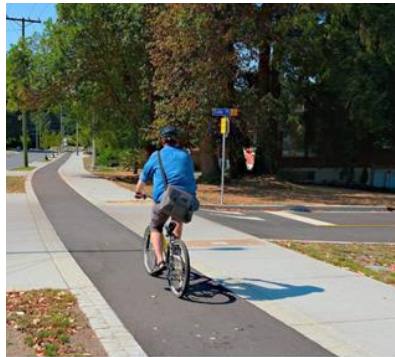
Continuous sidewalk/side-path trail.
