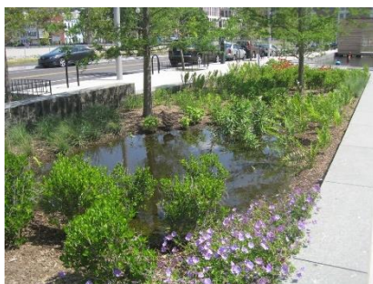
Rain garden (stormwater facility).
