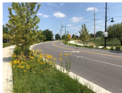
Bioswale (stormwater facility).
