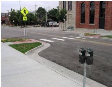
Curb extension speed management.
