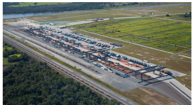
Central Florida Intermodal Logistics Center, Winter Haven.
