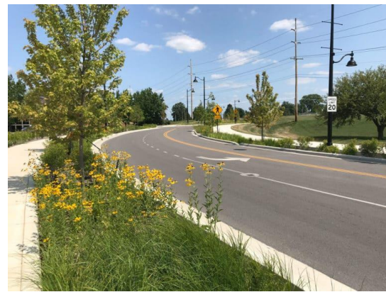
Bioswale green stormwater infrastructure.
