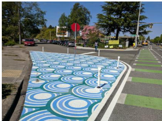
Daylighting with paint and flexible bollards.
