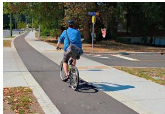
Sidewalk and trail at grade with driveway.
