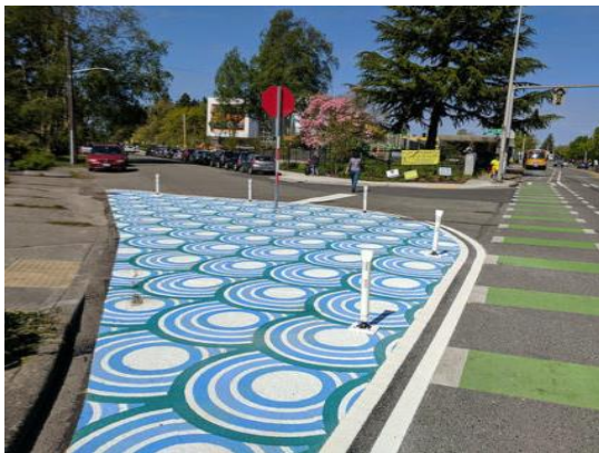
Daylighting with paint and flexible bollards.
