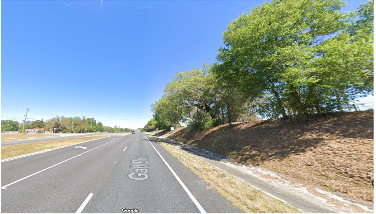
Photo 1 – Subject Site Viewed From Gall Blvd Looking Google Imagery -
