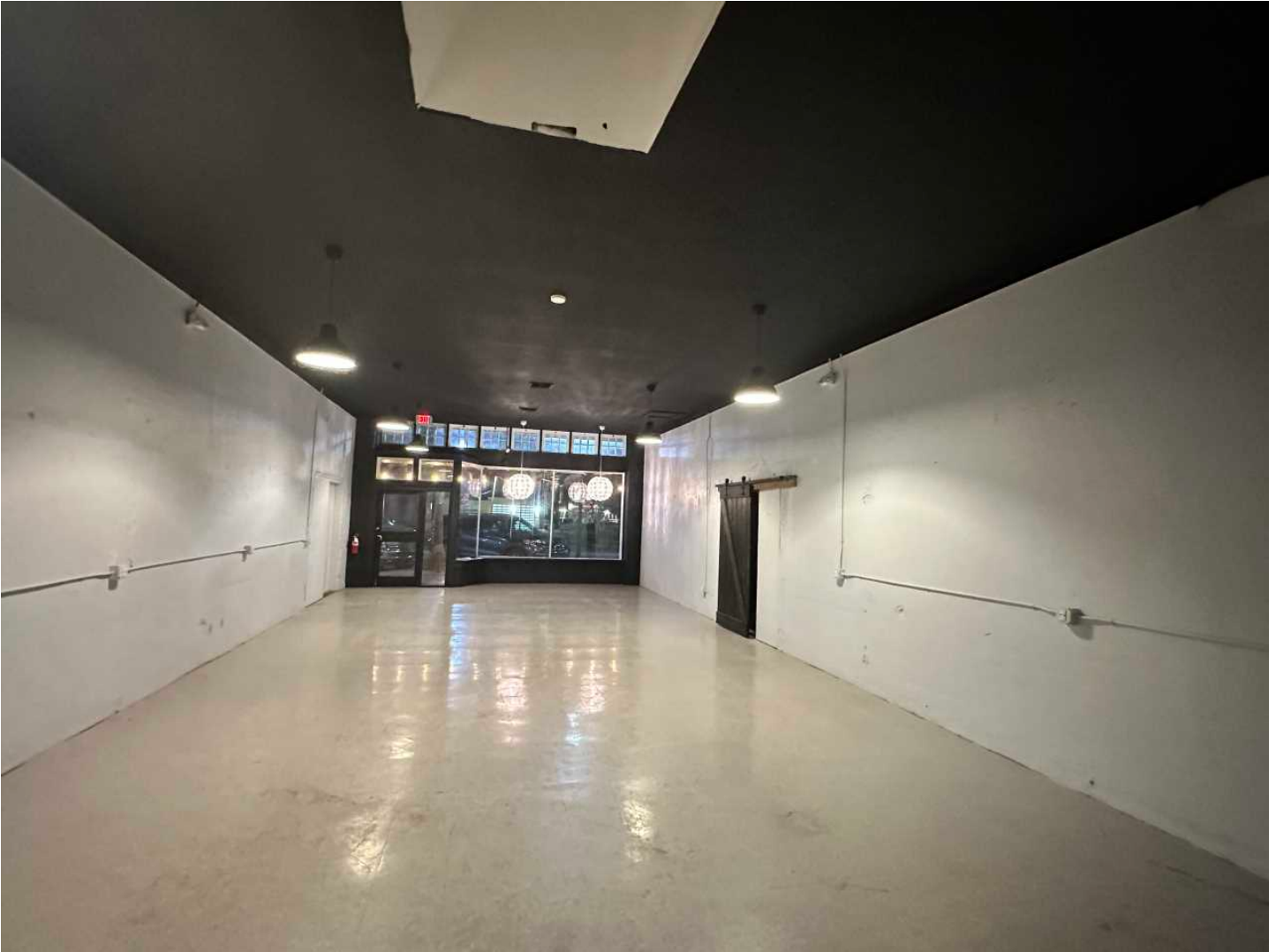
3 3-IMG_4408 Date Taken: 11/13/2024 Taken By: Wilman
