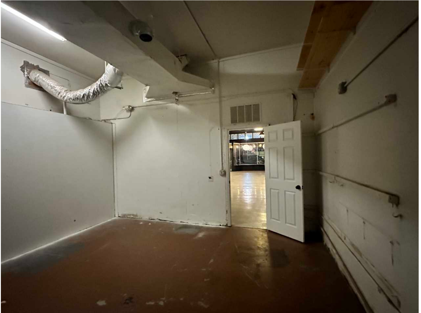
7 7-IMG_4412 Date Taken: 11/13/2024 Taken By: Wilman
