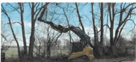
TIMBER LINE & FENCE ROW TRIMMING
