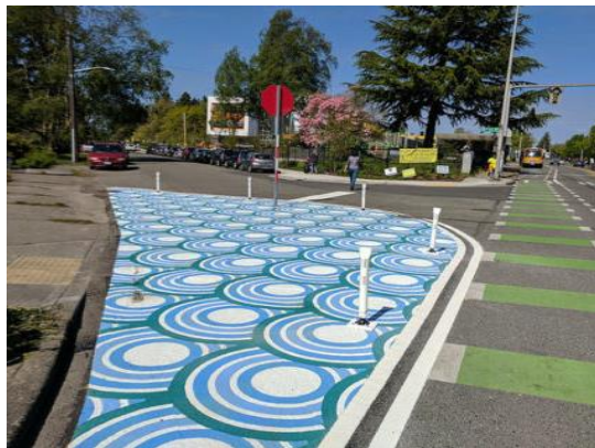
Daylighting with paint and flexible bollards.
