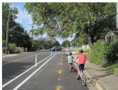
Separated (contraflow) bicycle lanes.
